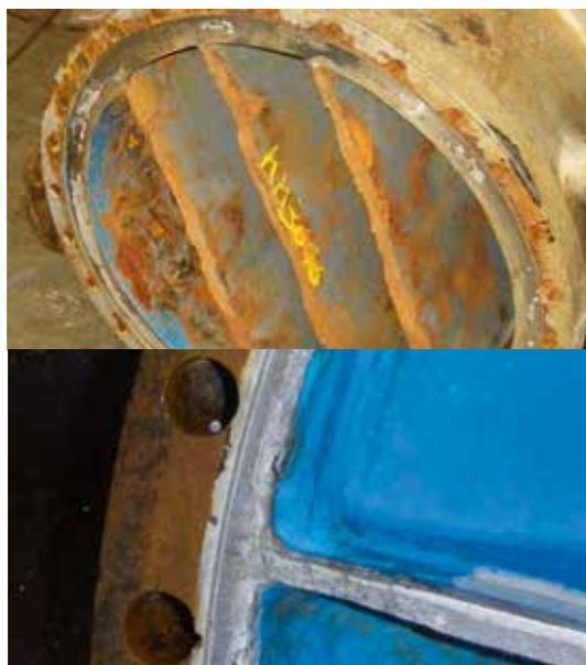
» Fig. 1. Some examples of corrosion issues on coated steel channels and floating heads. (Photo courtesy of TOTAL Antwerp.)
